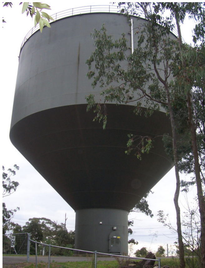
Figure 9 - Steel wineglass tank, 4ML storage capacity
