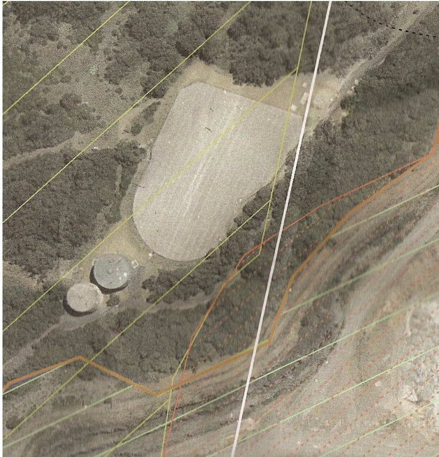
Figure 10 - Concrete in-ground tank, 38 ML storage capacity (note the two wineglass tanks adjacent)
